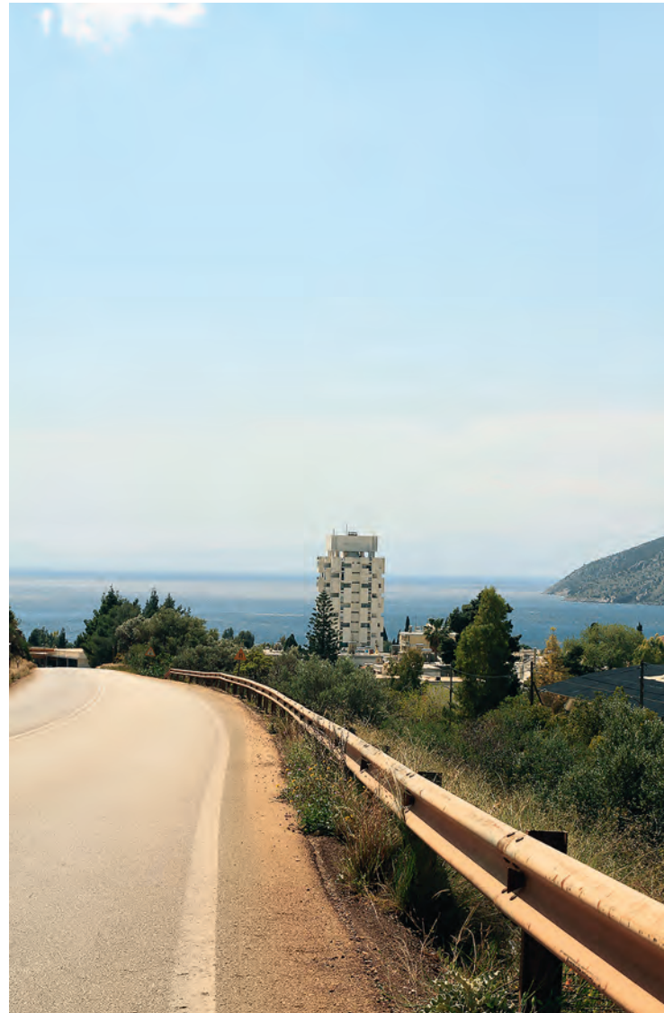
Fig. 2: Entering Aspra Spitia settlement, view of The Tower , 2024
